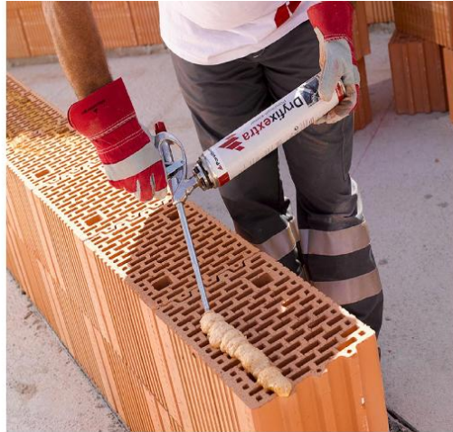
Slika 1: Porotherm 38 Profi opeka; Zidanje Porotherm DRYFIX sistemom (Wienerberger, 2017)
